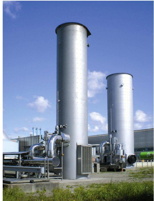
**Picture 2: HAASE sludge gas flares** Next to the flare operating since 2004 (left, 12,5MW), an additional flare was installed (right, 27MW). It is furnished with a two-stage burner and a pilot burner for midjet quantities
