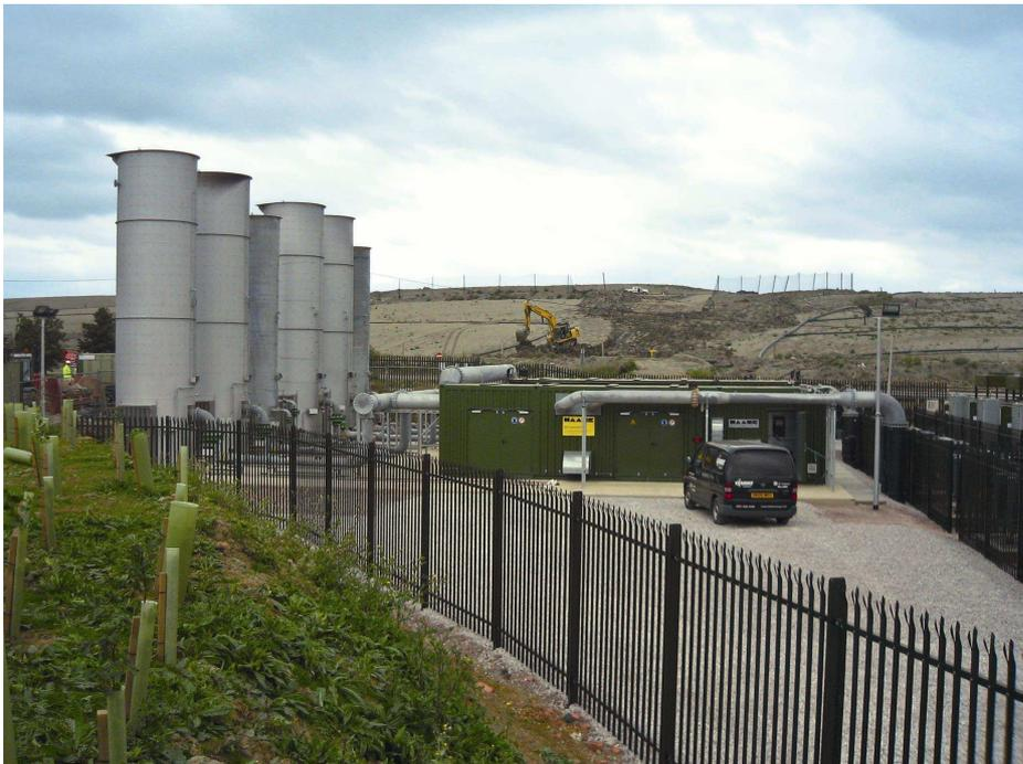
**Picture 3: 6 landfill gas flares on Brogborough landfill site, England** Total combustion capacity 100MW. The appending gas booster stations supply 27,6000m<sup>3</sup>/h of landfill gas
